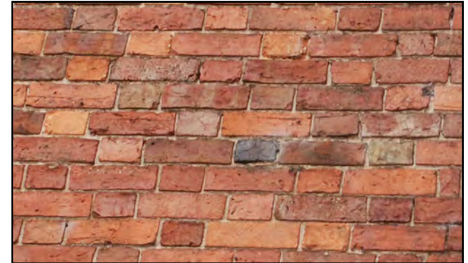
Reddish-plum brickwork of Georgian buildings
