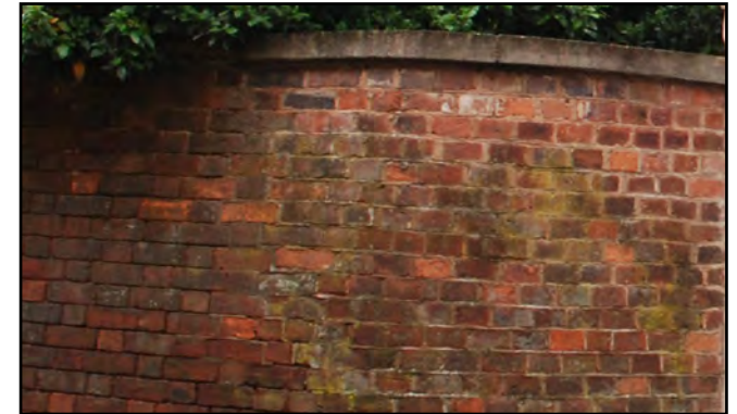
Low level red brick wall
