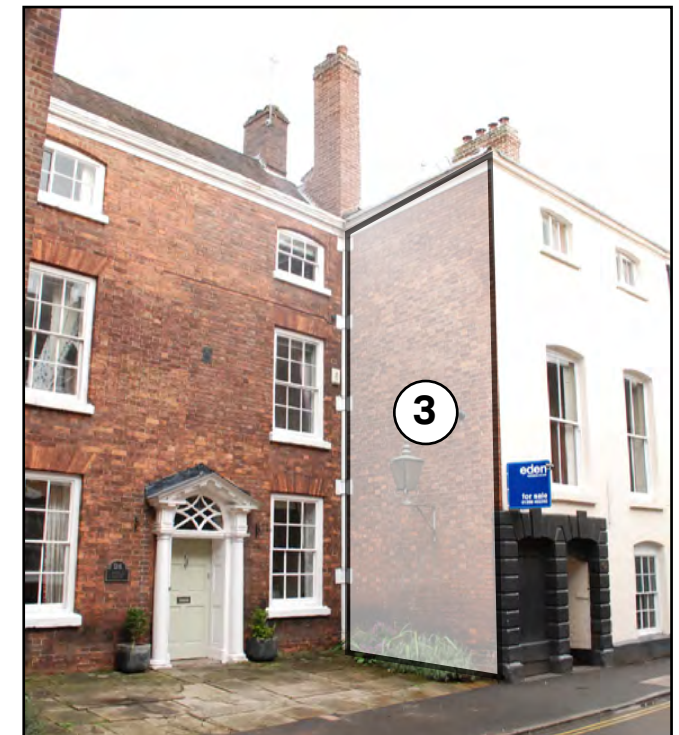
3- Recess in building line exposes gable ends and provides some set back from street
