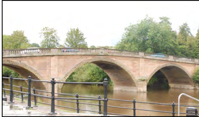
Bewdley Bridge- a Grade I Listed structure
