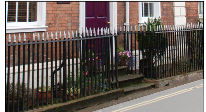
Iron fencing complements the Georgian facades
