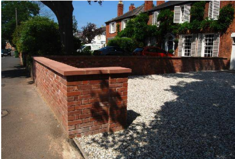
New wall built using traditional materials
