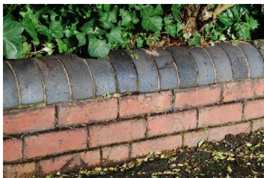
Historic dwarf brick wall
