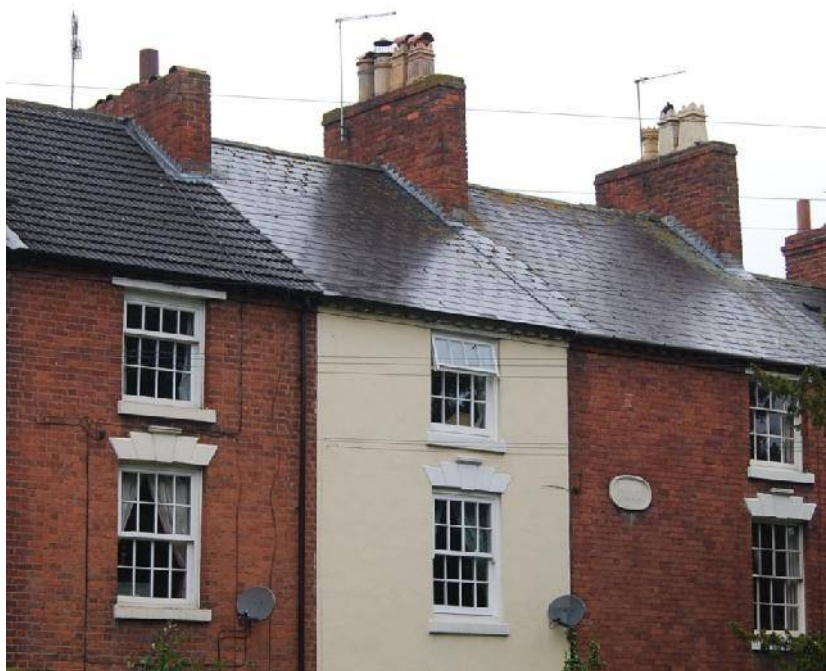
Comparison between concrete tiles (left) and slates (right)
