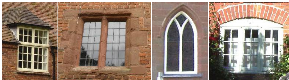
A selection of windows from within the Area
