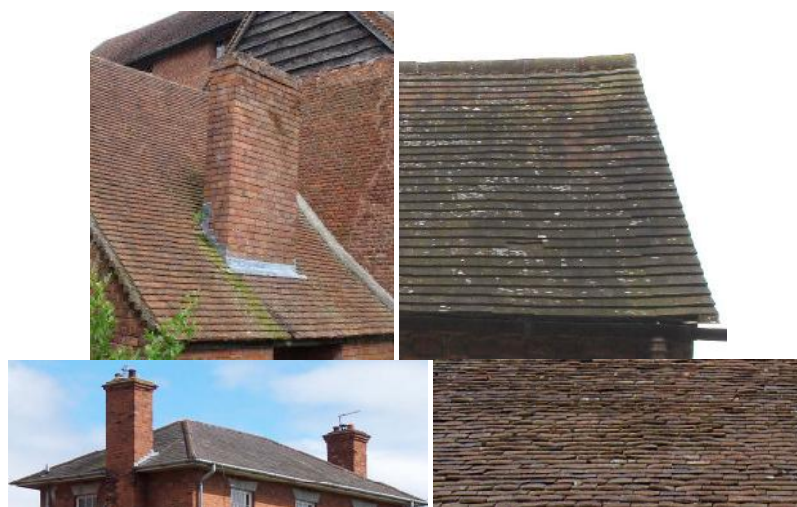
Examples of the roofing materials found within the Area
