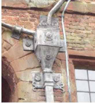
Lead downpipe and hopper at Harvington Hall
