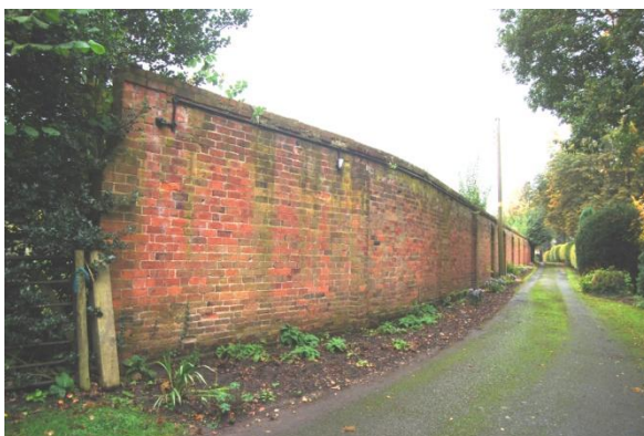
Brick wall to the rear of Areley Hall
