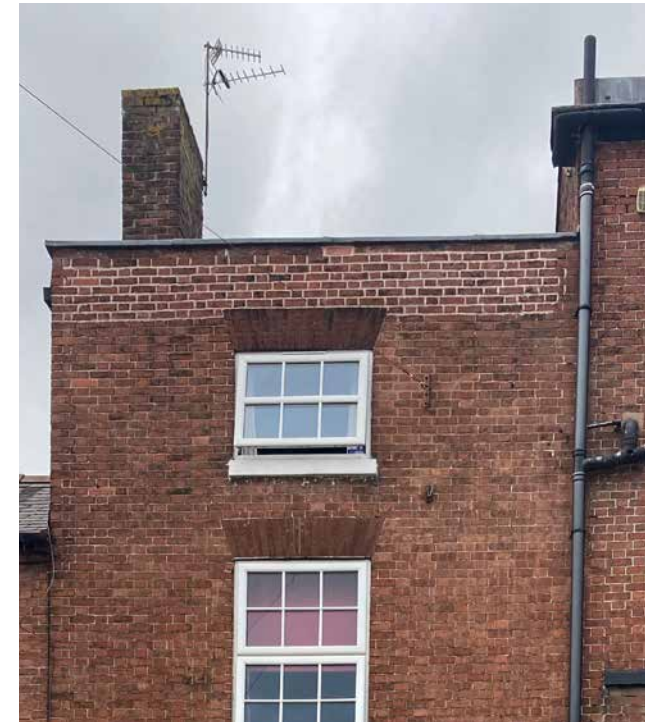
7.1 The use of inappropriate modern windows harms the appearance of buildings
