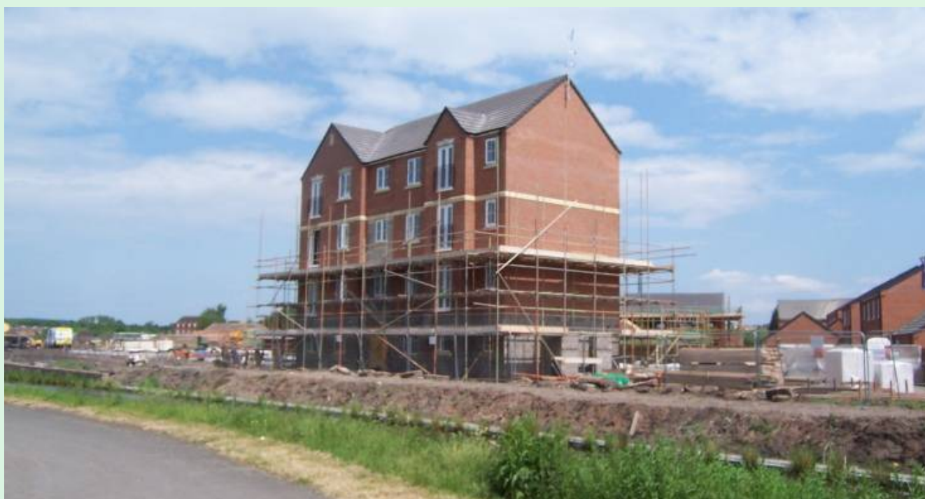
Canalside Apartments under construction, Churchfields
