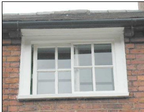
A rare horizontally sliding window, occasionally found lighting the upper storey
