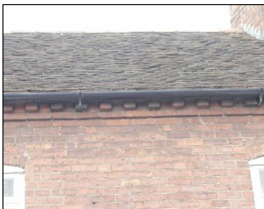
High quality parapet (top left) and eaves treatment (top right) and modest eaves treatment with hit and miss header dentilling (bottom left) and saw tooth dentilling (bottom right)
