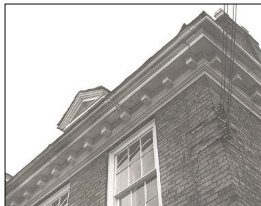
Pitched roofs with a frontal parapet (left of centre) and hip with eaves (right of centre)
