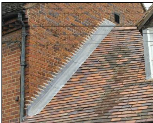
Lead flashing stepped with the mortar courses
