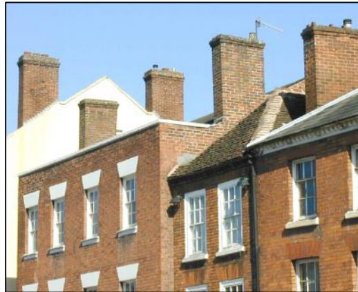
Pitched roofs with a frontal parapet (left of centre) and hip with eaves (right of centre)
