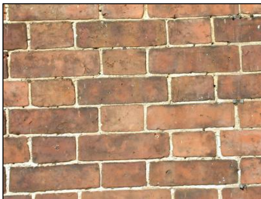
Brickwork with a traditional Flemish bond
