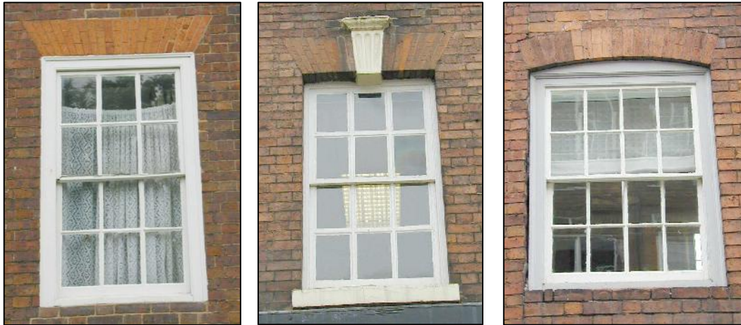
Close up of a front mounted sash window with gauged voussoirs (left) recessed sash window with gauged voussoirs, keystone and stone cill (middle) and front mounted sash window with segmental brick header (right). Note that each voussoir to the flat headed windows is individually gauged and of a finer grain and quality than the brickwork, and that front mounted windows have wide architraves
