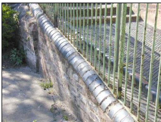
Traditional semi-circular coping to the top of a wall
