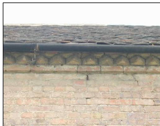
High quality parapet (top left) and eaves treatment (top right) and modest eaves treatment with hit and miss header dentilling (bottom left) and saw tooth dentilling (bottom right)
