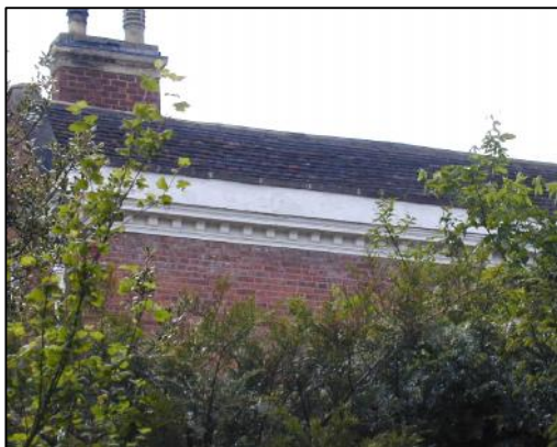
Pitched roofs with a frontal parapet (left of centre) and hip with eaves (right of centre)
