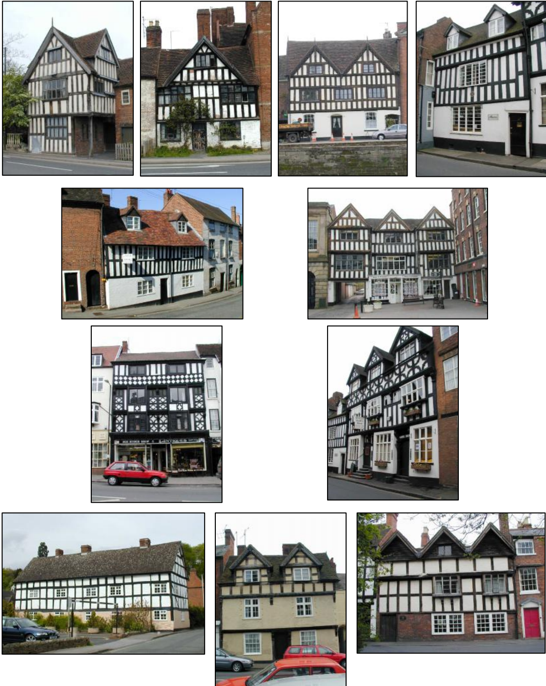
Variations of timber framing, with close studding (first and second rows), panels and quadrant braces (third row) and square framing (bottom row).
