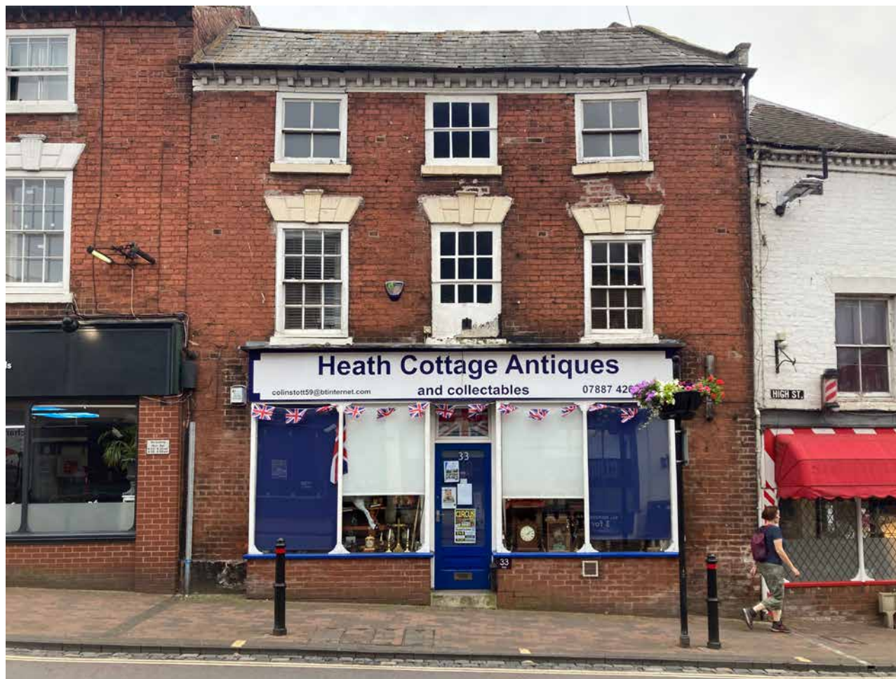
5.20 Blind windows (centre) with painted sashes. Painted brick dentil course at eaves level
