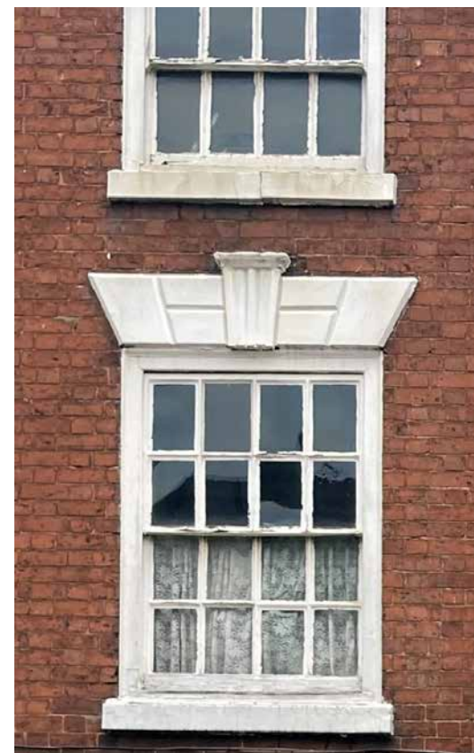
5.18 Sash windows with exposed sash boxes and voussoir arches with key stones
