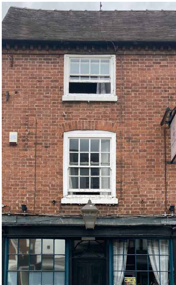
5.19 Sash windows in openings with segmental brick arches
