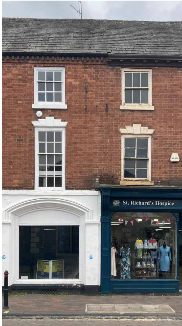
5.21 No party wall division at roof level. Note change in eaves level
