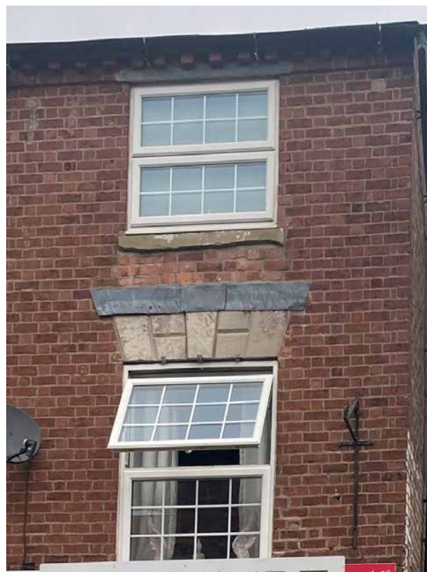
7.1 The installation of modern windows of inappropriate design harms the conservation area
