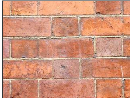
Brickwork with a Flemish bond
