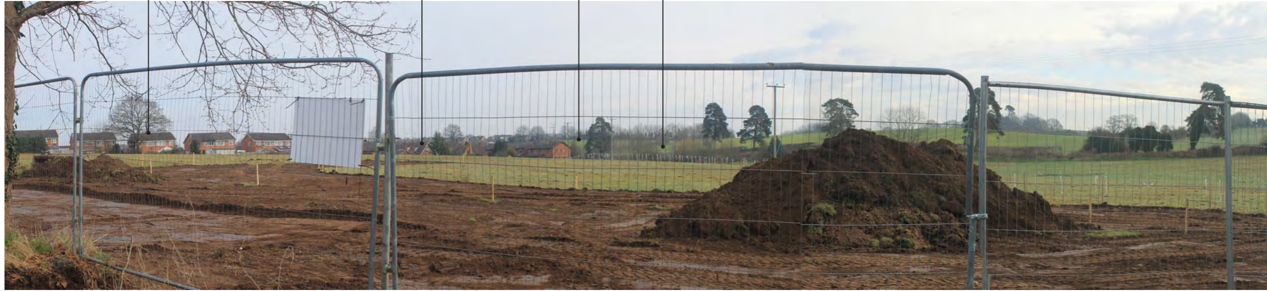
Photograph 23 View from Pearl Lane B4194, looking north east towards Site.
