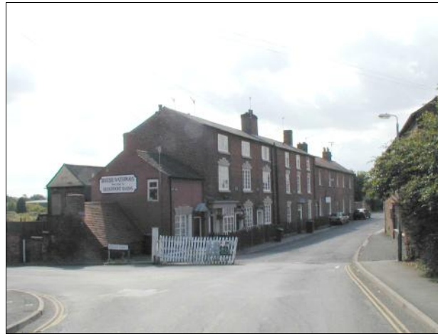
Terraced houses in Mart Lane
