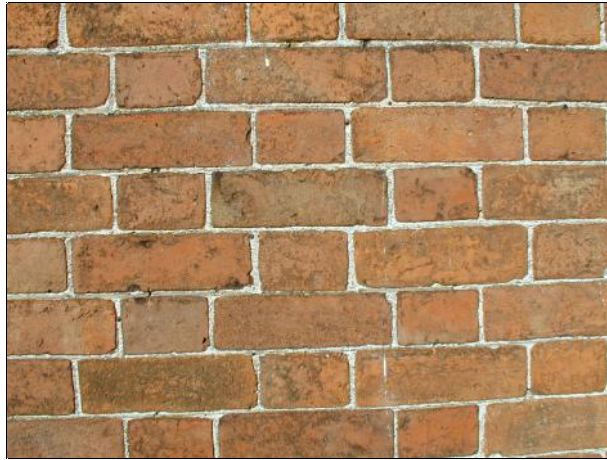
Brick-work with a traditional Flemish bond
