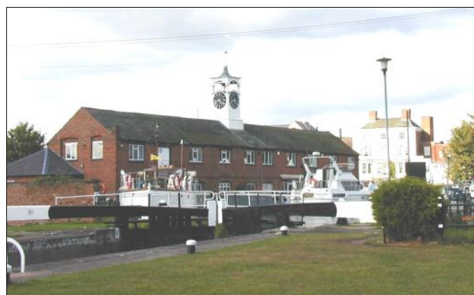
Former warehouse at the centre of the basins, now occupied by Stourport Yacht Club
