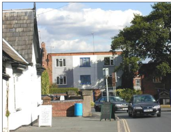
View looking east along York Street towards unsympathetic flat roofed houses in Lion Hill
