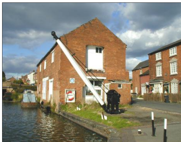
Former warehouse and adjoining crane in Mart Lane
