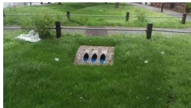
Concrete pipe surround has been used here to provide minimal cover for a driveway crossing at Devonshire Hill, Haringey.
