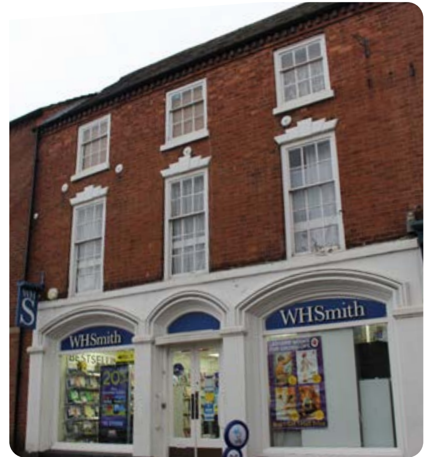
Red brick is the predominant building material. Doors and windows have a strong vertical emphasis.
