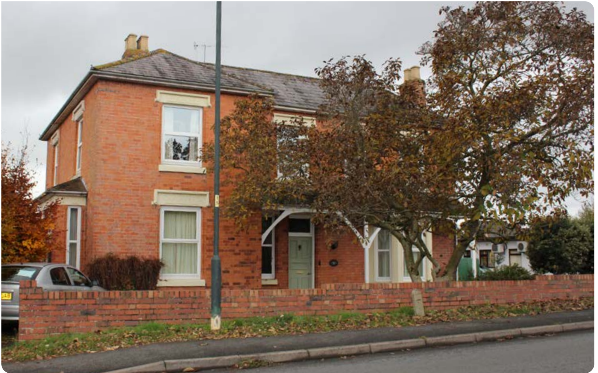
An example of a building with orange and red brickwork in Flemish bond and low cross hipped roof.
