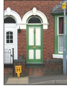
A selection of mid. to late nineteenth century doorways found within the Area. Note the door to the left (with large window) is a modern replacement, and the doorway in the centre may be a Victorian remodelling of an older building
