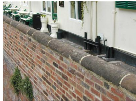
Walls with traditional semi-circular blue coping (left) and sandstone coping (right)
