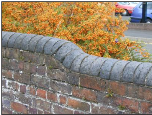
Walls with traditional semi-circular blue coping (left) and sandstone coping (right)
