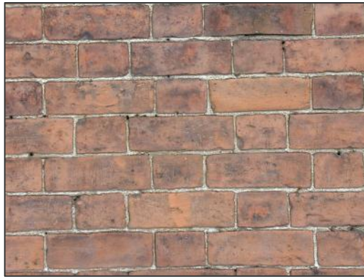
Brick-work with a traditional Flemish bond
