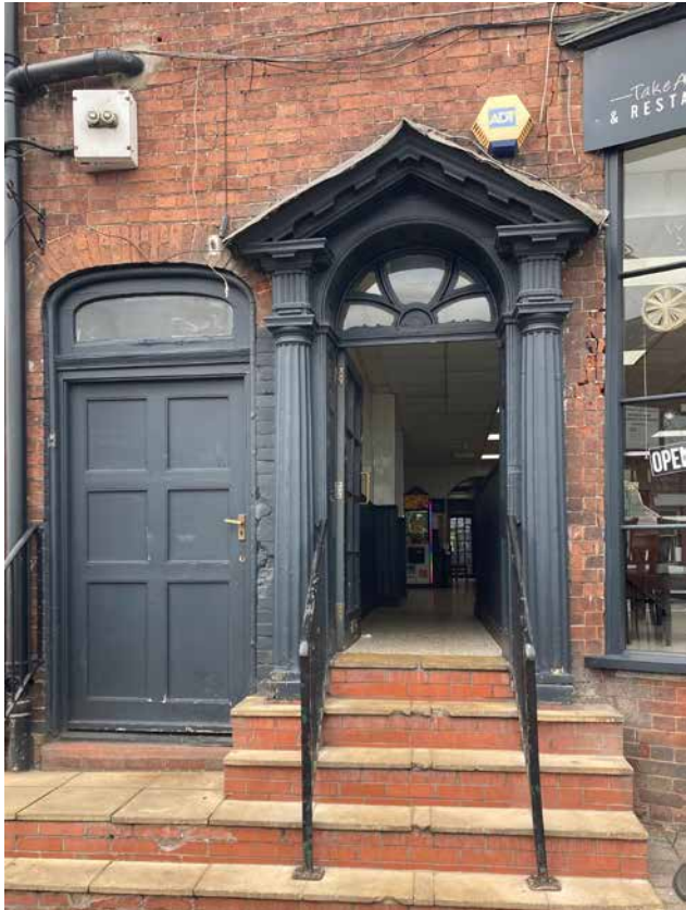
5.23 No. 13 Bridge Street. Entrance to house and passageway (left)
