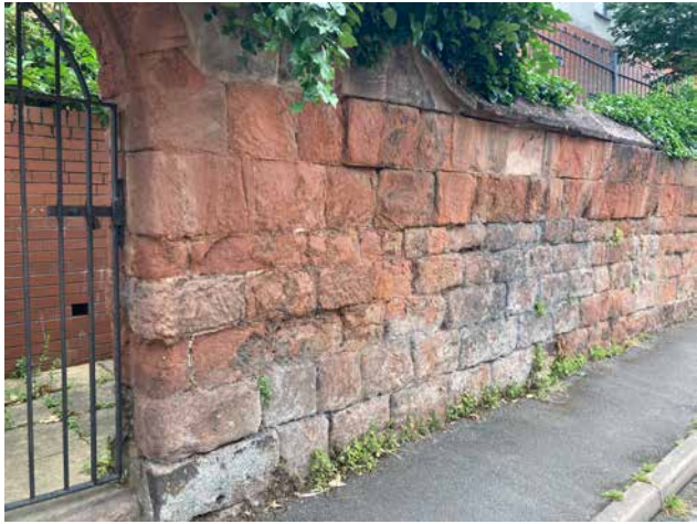
5.25 Cheapside - East wall to Lichfield Basin
