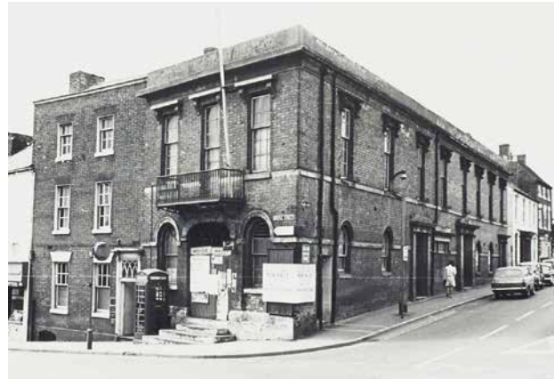
3.8 Old Town Hall, built in the 1830s, collapsed 1973 (Worcestershire County Archives and Kidderminster Shuttle)
