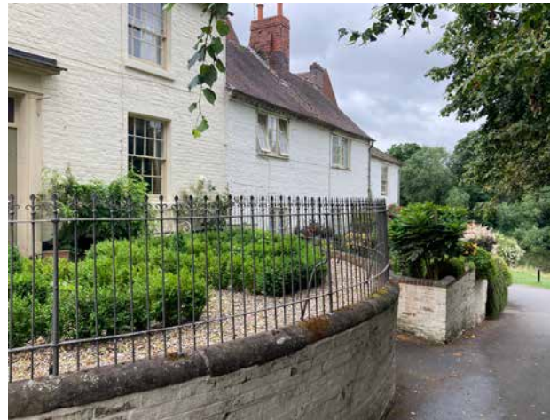
8. Severn Side - Nos. 1, 2 and 3 (early 19C)
