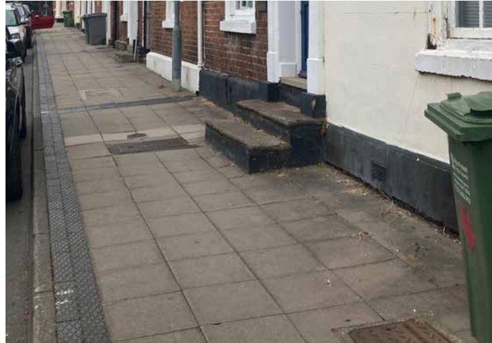
5.28 Bridge Street - modern brick paving
