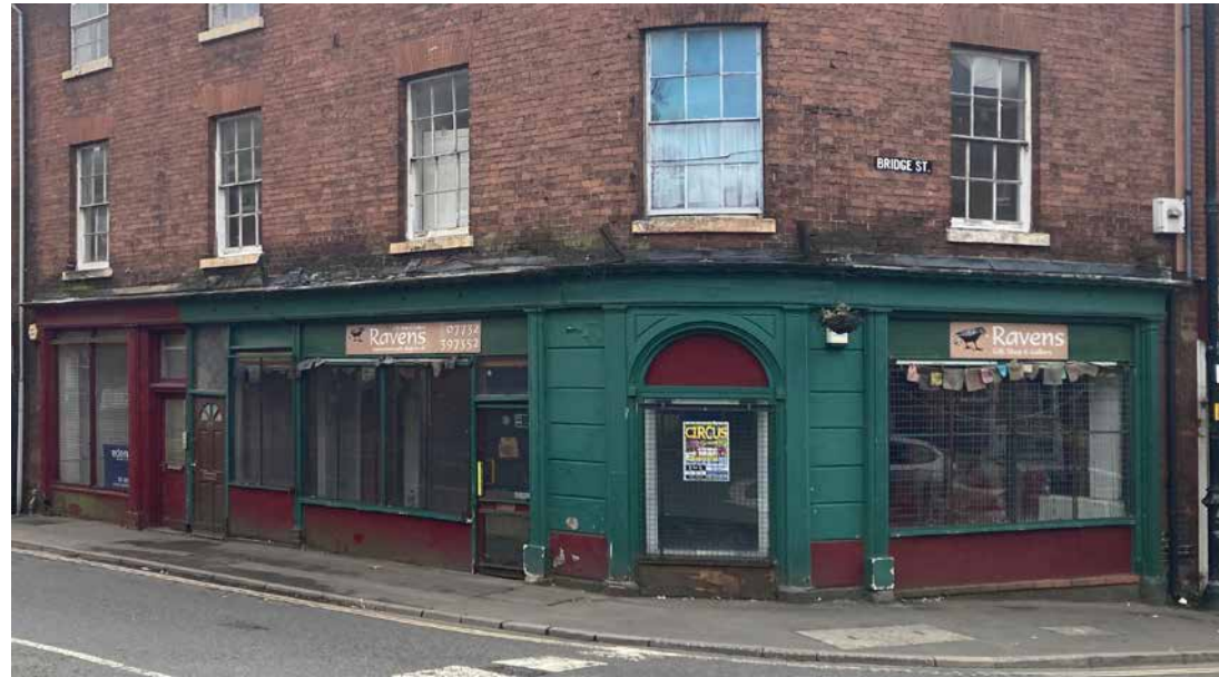
10. York Street - Nos. 22-24. A Georgian framework of pilasters and fascia, with modern shopfront within
