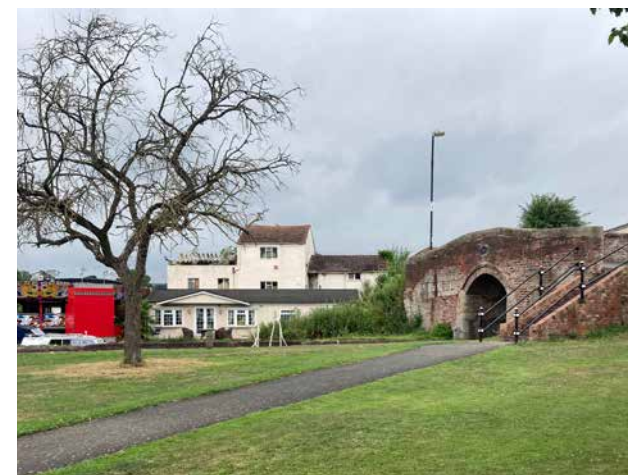
1. The engine house (middle) and bridge over the channel
