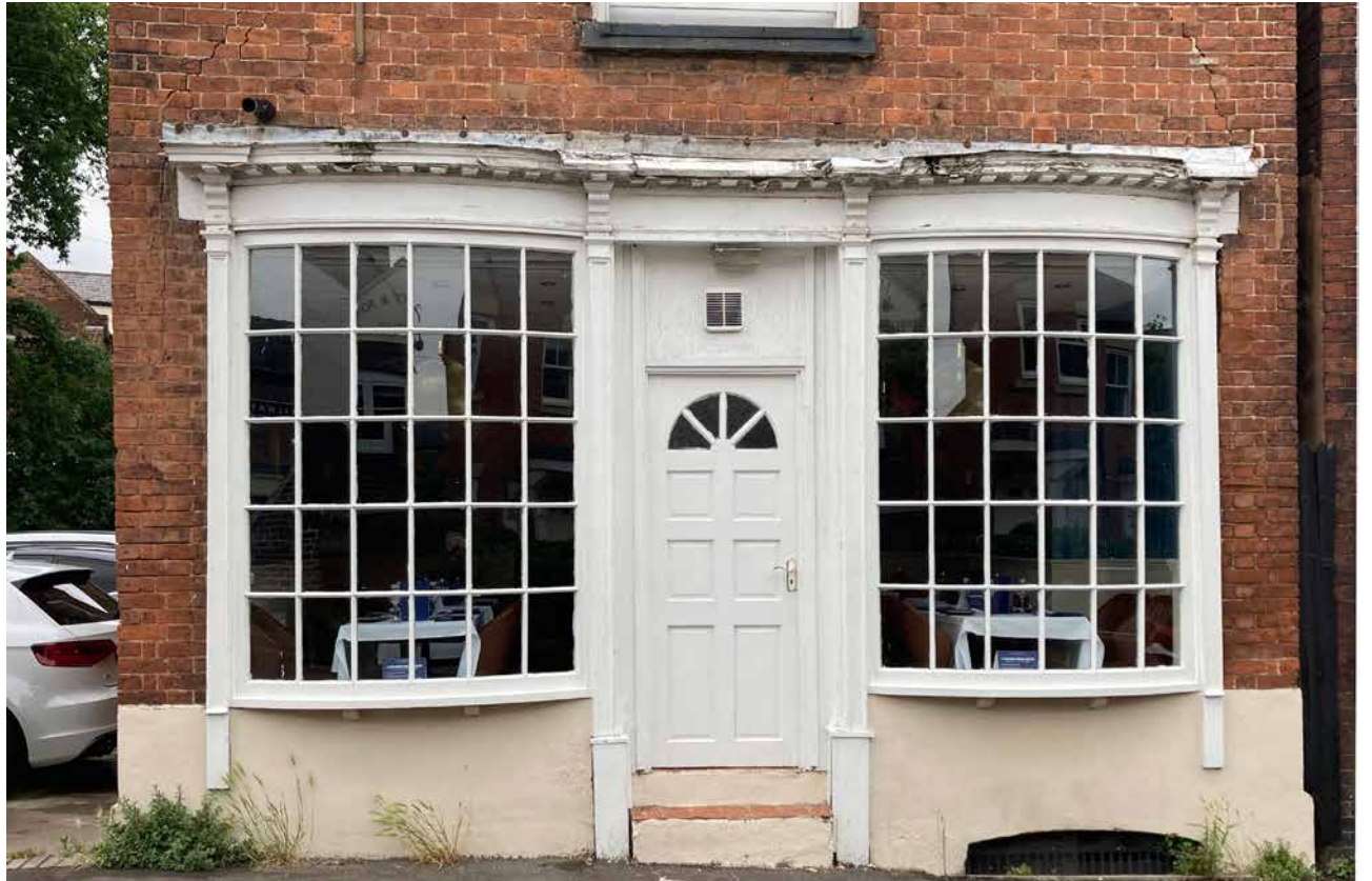
5.24 No.1 Lichfield Street. Symmetrical early 19C shopfront
