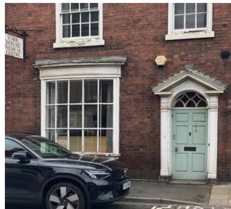
9. York Street - No. 20 with Georgian shop window
