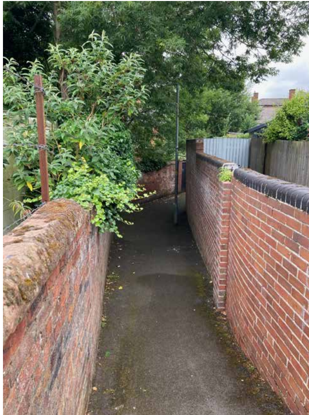
5.26 Brick walls lining the passageway from Severn Side to Cheapside
