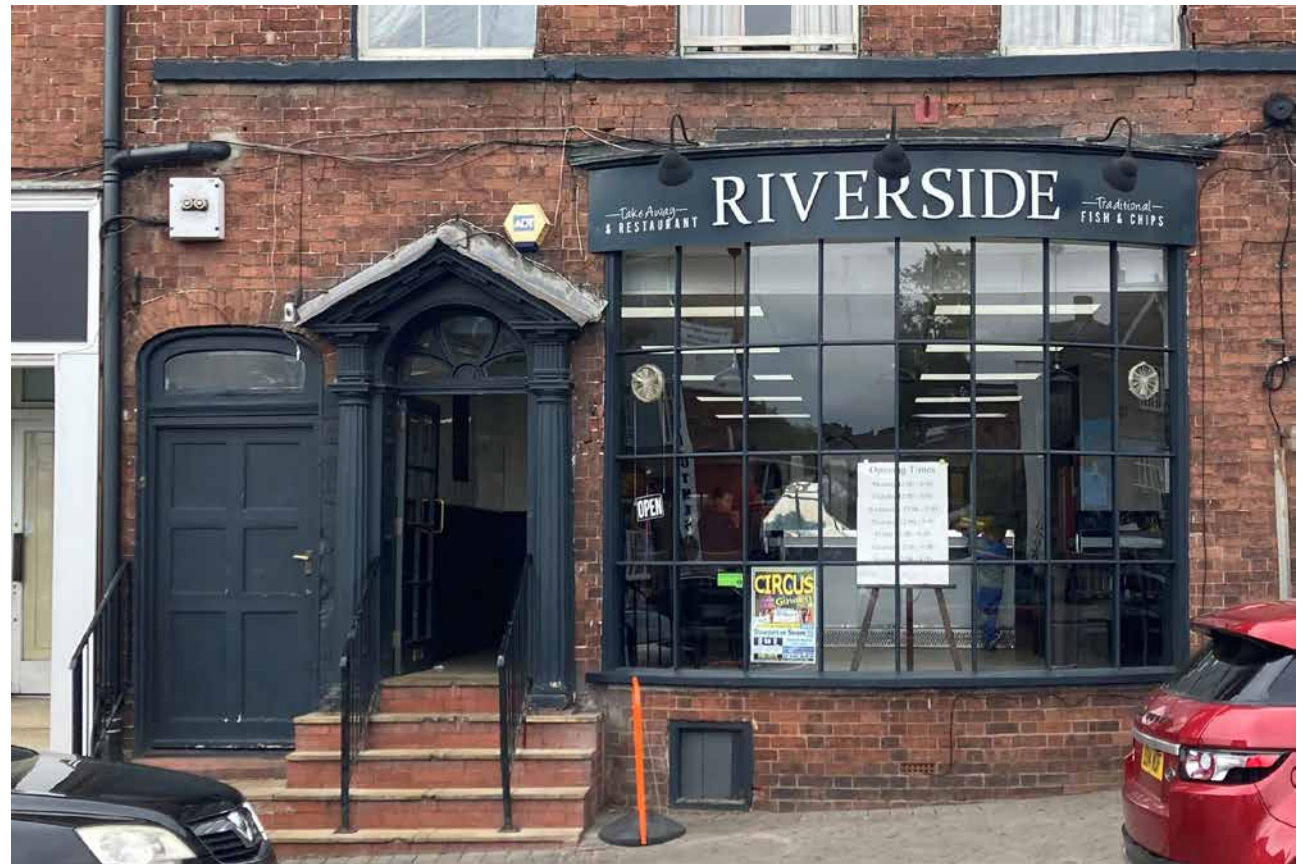
1. Bridge Street - No. 13. A Georgian style shopfront
