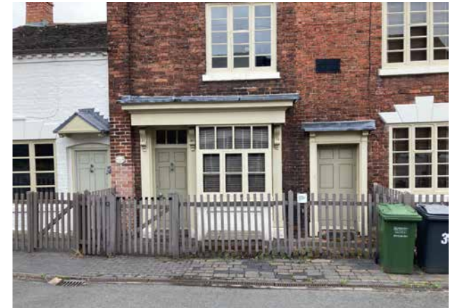
5. Mart Lane - No.2. An altered 19C shopfront
