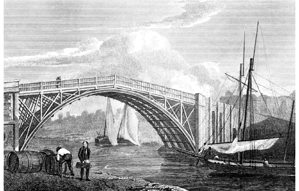
3.7 Stourport's iron bridge, built in 1806 (1812) (H68XAR (002)) (Alamy)
