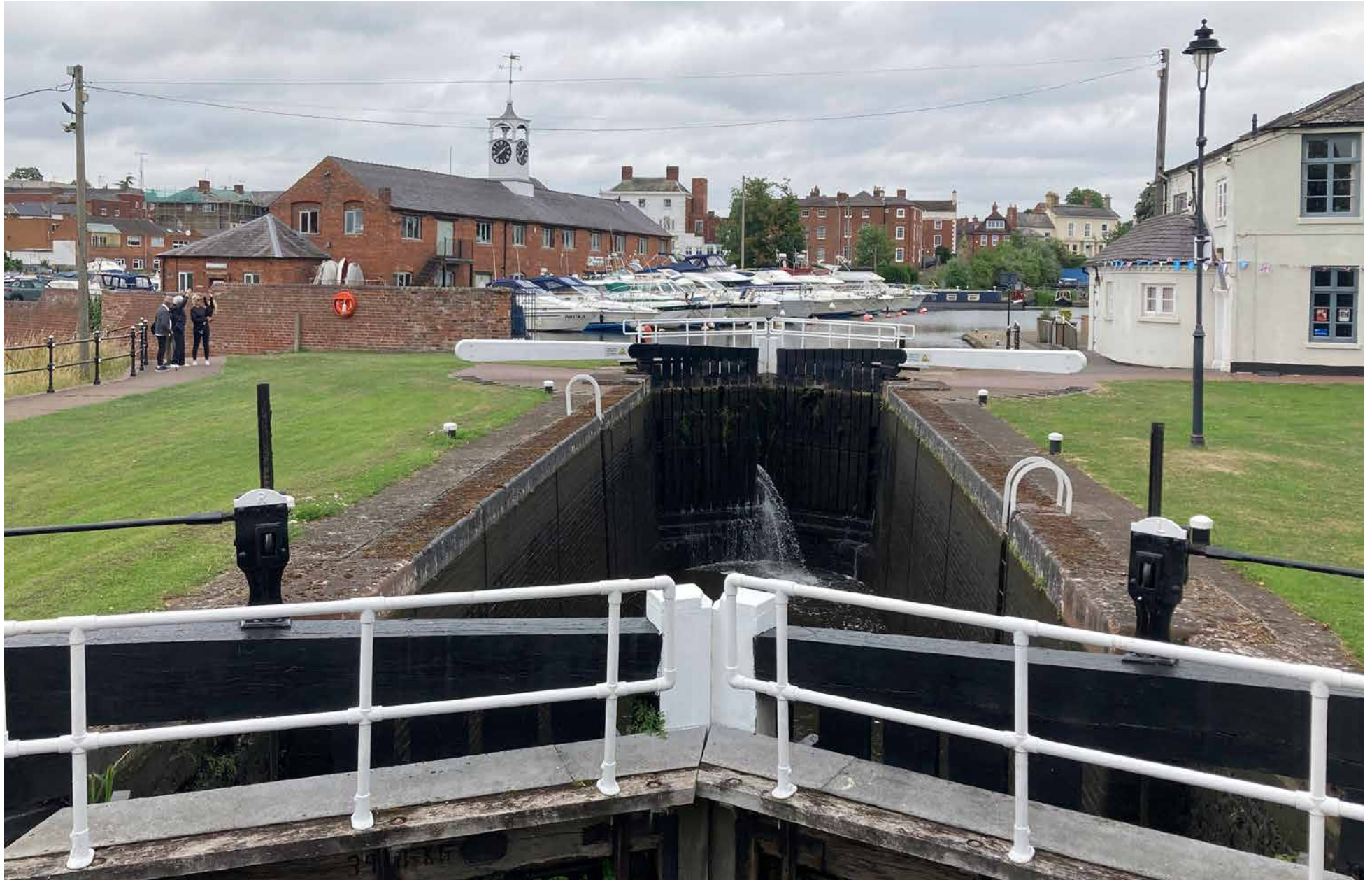
1.2 View across the Upper Old Basin towards York Street. The Clock Warehouse is on the left. The former Iron Warehouse is on the right.
