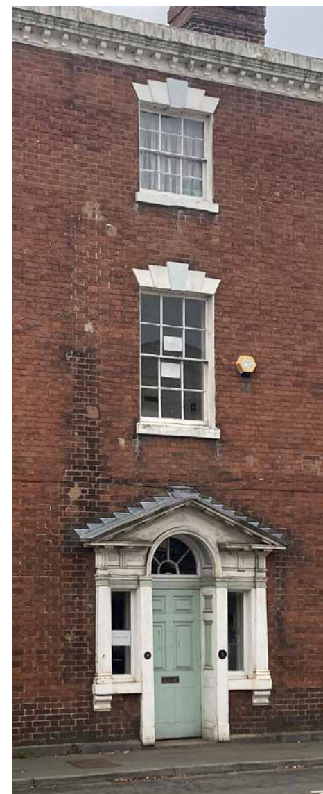
6.1 Part of the facade to York House, York Street
