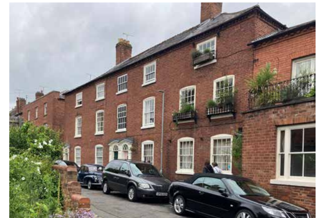
6. Lichfield Street - Nos. 5 to 8 (right) (early 19C)
