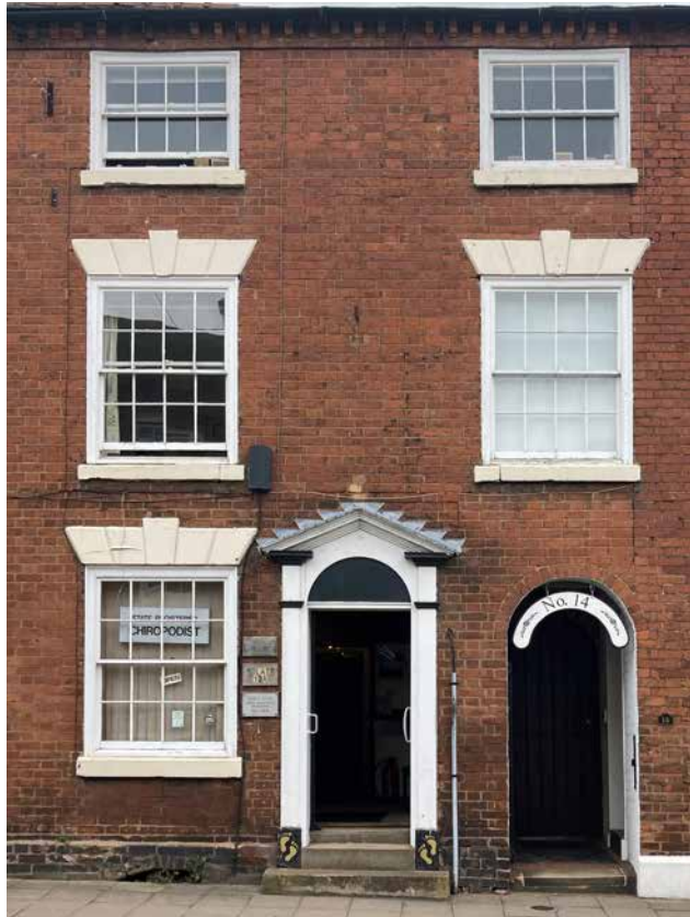
5.20 New Street facade
